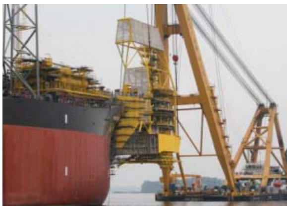
Lifting and integration of the turret to the FPSO
