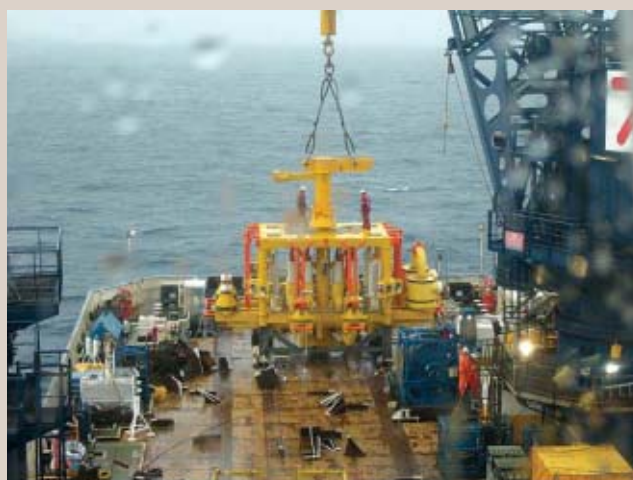
One of 5 Aker Kvaerner Subsea manifolds being installed.
