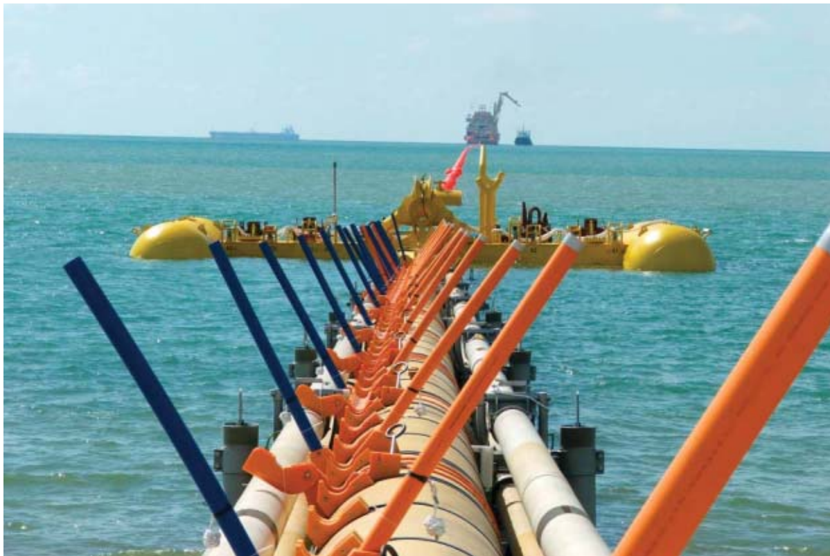
The FTL being towed onto sea surface using the Normand Installer
