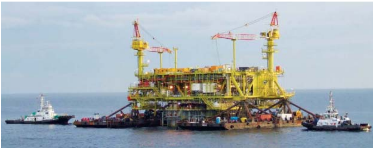
The topside being prepared for transfer onto the Spar hull via a float-over technique
