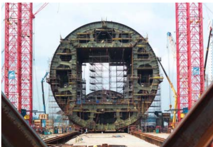
Construction of the Spar hull underway in Pasir Gudang, Johor
