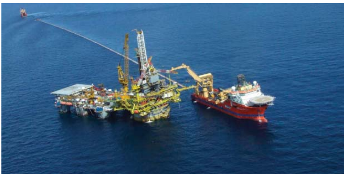
Kikeh's FTL is the first in the world that uses gravity actuated pipe (GAP) technology
