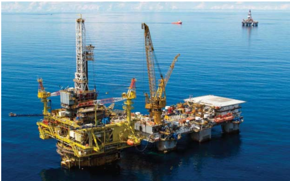
West Setia, a semi-tender assist drilling rig, will drill and complete 18 wells from the Kikeh Spar
