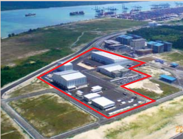
Aker Kvaerner's purpose built $100 million subsea equipment facility in Port Klang, Malaysia.
