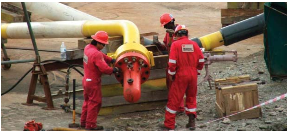
The flowlines were fabricated using quality pipeline fabrication methods
