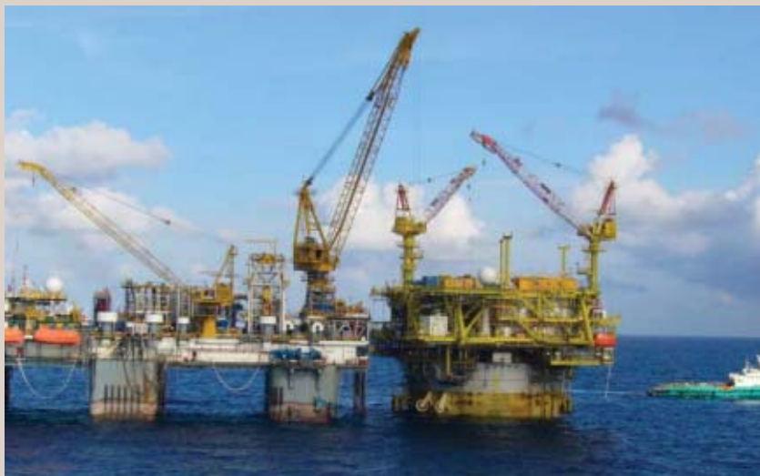
The tender assisted rig hooked up to the dry tree unit (spar).
